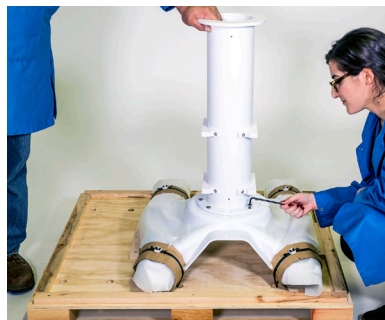
Install column with 8 M8 screws.
